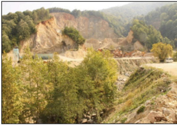
Quarry near Yanık Creek and the dumping of debris into the fish habitat (Original).
