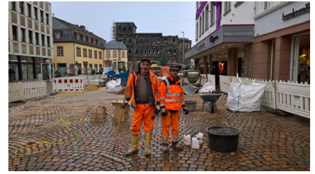
Figure 26 Paving masters and the Calçada Portuguesa, Trier ©MJ Duran Kremer.
