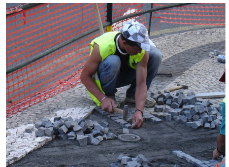
Figure 4 Laying the pattern ©Zureks.
