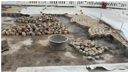
Figure 7 Laying the pavement, Trier ©MJ Duran Kremer.
