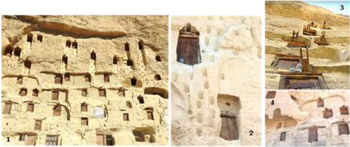
Resim 11. Taş ambarlar, tutamak, sekemek, kapı ve makara örnekleri (Photo 11. Stone warehouses, holdings, bins, door and drum samples)
