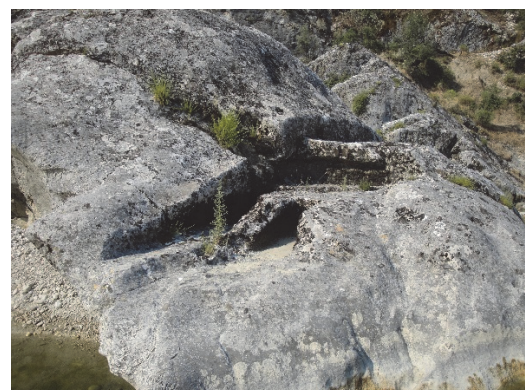
Fig. 18) Western footing of the wooden bridge
