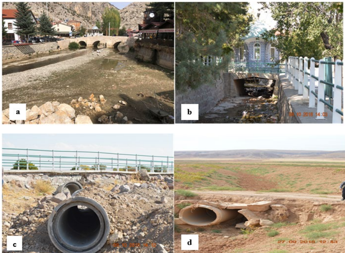
Figure 6. Narrowing the flood protection structures by construction of infrastructures (a) Konya Bozkir district, b) Konya Yarasli region, c) Konya Yarasli Region, d) Konya Kutukkusagi Region)
