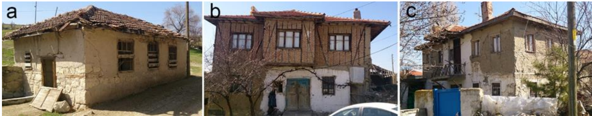
Sekil 3. Examples of masonry stone, masonry Adobe and wood carcass brick infill structures
