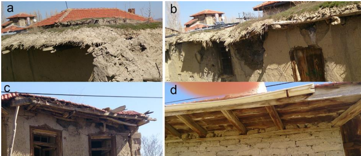
Figure 6. Photos on top cover: earthen dam (a, b); gable roof (c, d)
