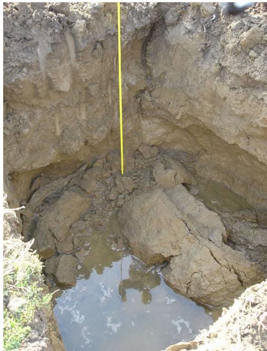
Figure 9. A view of a selected soil investigation trench showing running sands due to water flow.
