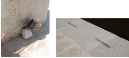
Figure 6. Stones and lead castings connected with sutures, Saraçhane Bridge repair
