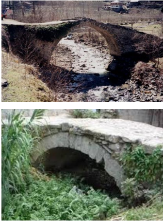
Figure 10. Kinali bridge and Ozbek bridge
