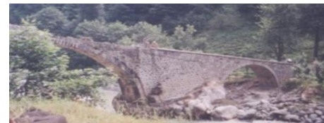
Figure 17. Repair works at Orenkit Bridge [4]
