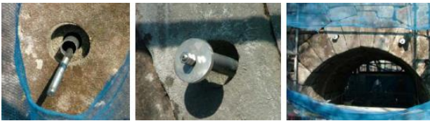
Figure 14. Horizontal anchorage application [15]
