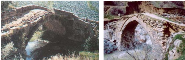
Figure 11. Historical Hersan and Ilicak bridges in Bitlis
