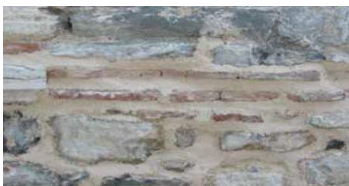
Figure 15. Reconstruction of the demolished part with mortar
