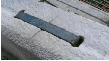
Figure 13. Use of steel tenon
