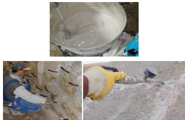
Figure 12. Injection application
