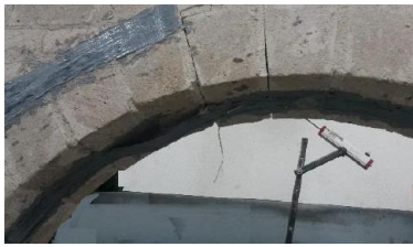
Figure 18. FRP strengthening [9]
