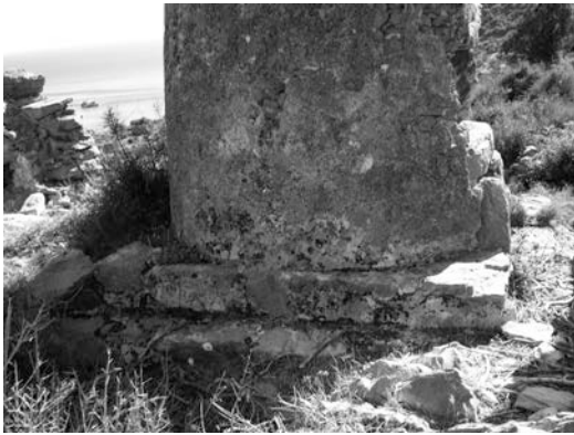
Fig. 21. Base of conical section of tower from the north
