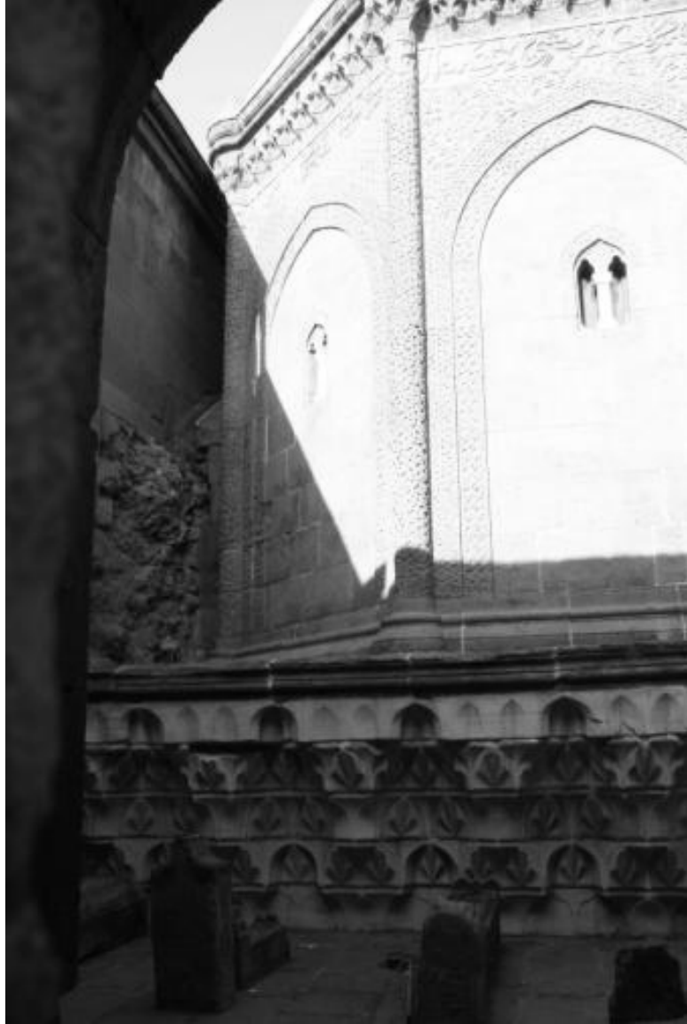
Figure 5: Huand Hatun Complex, Kayseri, view on mausoleum from the entrance corridor of the mosque (photo: author)
