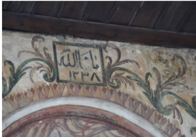
Visual 3. Inscription on attic plaster on the entrance door of narthex in Ethem Bey Mosque
