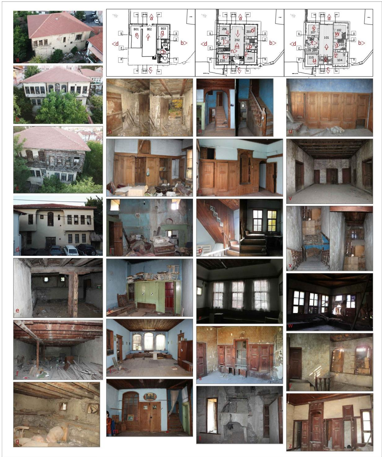
Figure 4. Photographs of Uşakizade Rıfat Edendi Mansion (2020)
