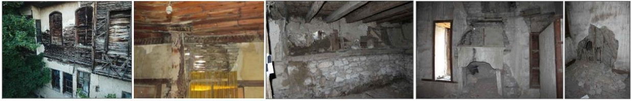
Figure 6. The construction technique used in Uşakizade Rıfat Efendi mansion
