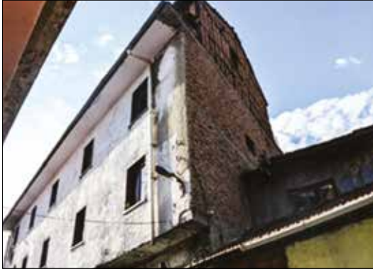
Fotoğraf 18: Rençber Han ön cephe / Front facade of Rençber Khan
