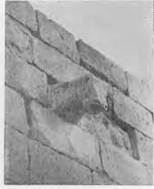
Res. 29a, b — Kayseri Sahip ata Medresesi çörtenci. Figs. 29a, b — Gutters at Sahip Ata Mcdrese, Kayseri.
