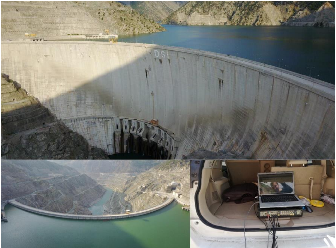
Figure 1. Some photos of the experimental measurements carried out in Deriner Arch Dam.
