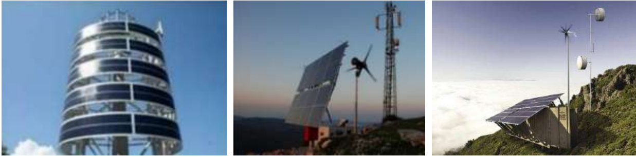
Figure 12. Various ways to find electric power to cellular base stations [65]
