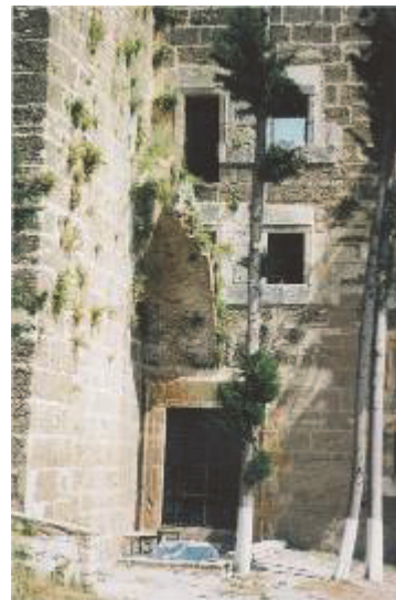
Fig. 12: General view of this façade.
