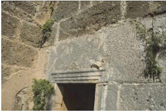
Fig. 14: The indications and in situ remains of the two roofs remaining on the lintel.
