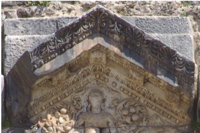
Fig. 28: The remains of stucco infilling in the border to the tympanum and around the head together with surrounding bullet marks.
