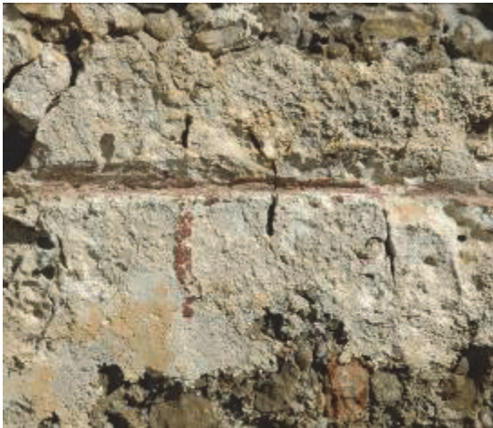
Fig. 26: Areas of yellow paint and red painted stone block outline on the block adjacent to the end of the upper row.
