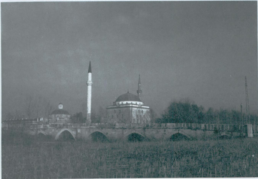
Fig. 24 — Yeni İmaret (Bayezıt) bridge.
