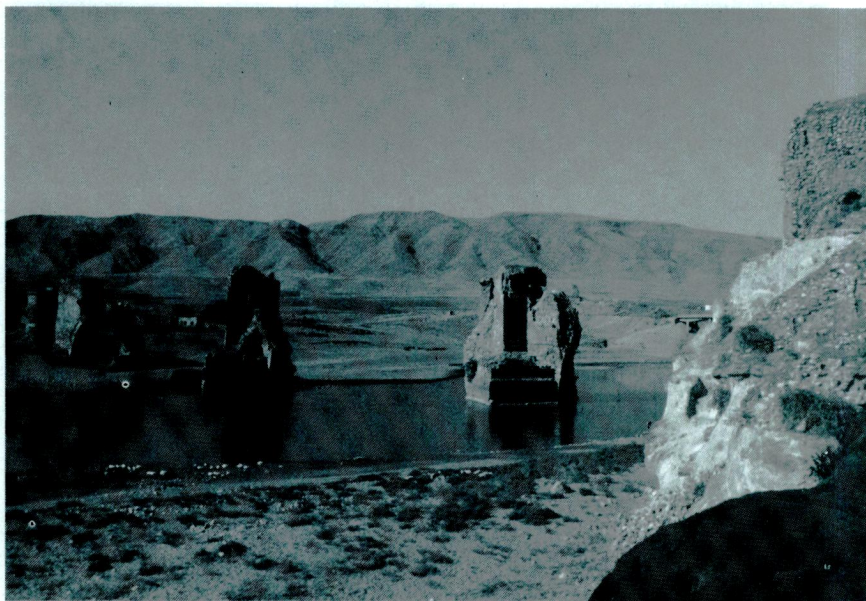
Fig. 13 — Hasan Keyf bridge.
