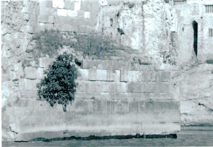
Fig. 16 — Hasan Keyf bridge.
