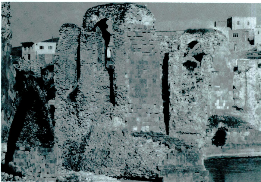
Fig. 14 — Hasan Keyf bridge.
