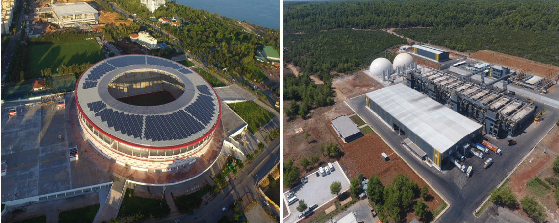
Figure 10. Antalya Stadium and Antalya Solid Waste Integrated Assessment Recycling and Disposal Facility [19]
