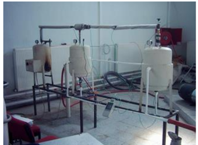
Figure 6. A photograph of experimental steam ejector cooling system
