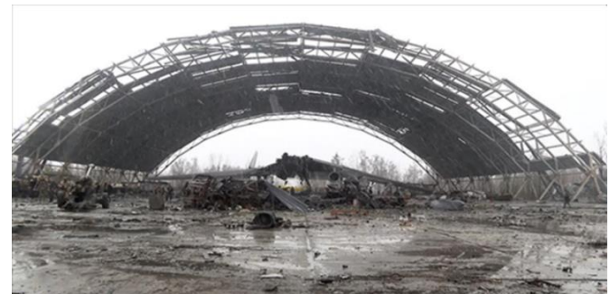
Figure 10. The final state of AN after the attack (NTV,2022)
