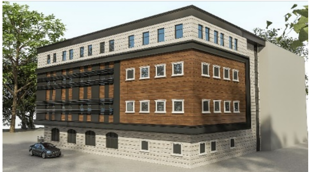
Figure 18. Kars Land Registry and Cadastre Directorate New Service Building (Çelik's personal archive)
