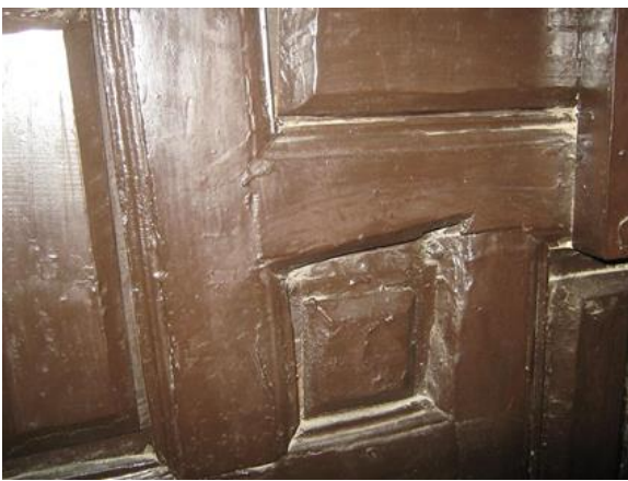
Figure 7. Details from the women's gathering room where coating was applied.
