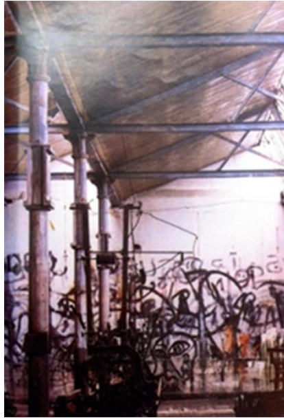
Figure 3. Feshane-i Amire before the first restoration [27]
