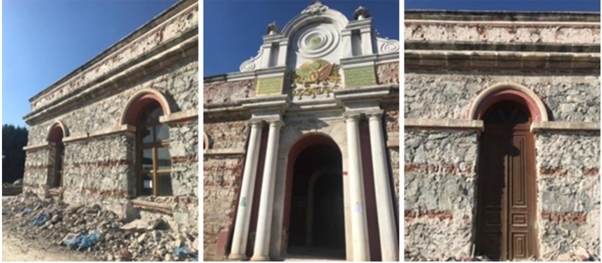
Figure 7. Currently exterior masonry wall
