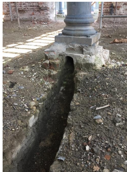
Figure 12. Detail of the column drainage system before it was covered
