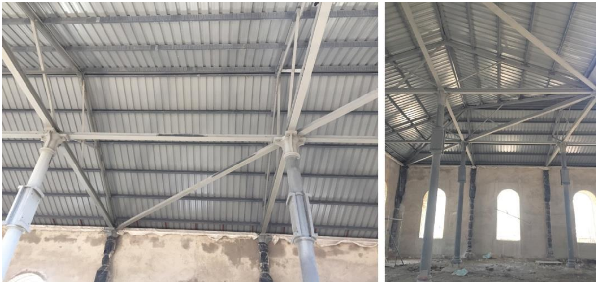
Figure 10. Currently roof trusses and braces
