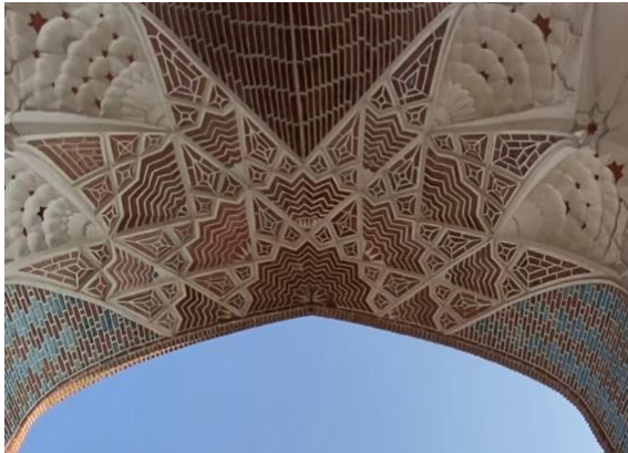
Fig. 24. Mogharnas of the entrance porch (Iwan) of the Akbariyeh School (Photo by: Authors, 2022)
