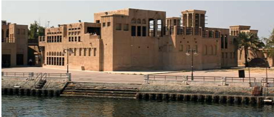
Figure 6: Exterior view for Sheikh Saeed Al Maktoum house (URL-5)
