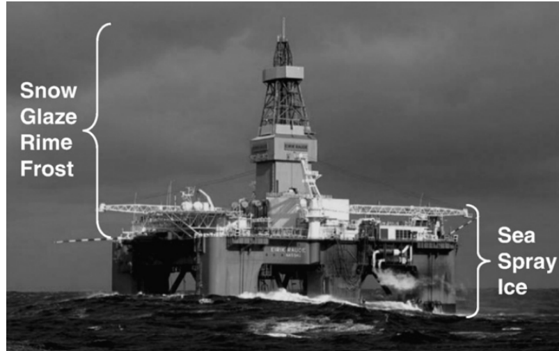
Figure 3. Icing effects on offshore structures [15].
