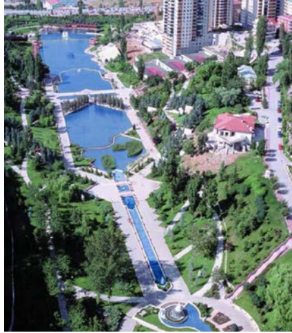
Figure 3. A view from Dikmen valley housing and environmental development project (Demirci, 2004).
