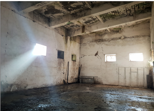
Fotoğraf 5. Z01 no.lu mekan (Ambar-1) / Room Z01 (Warehouse-1).
