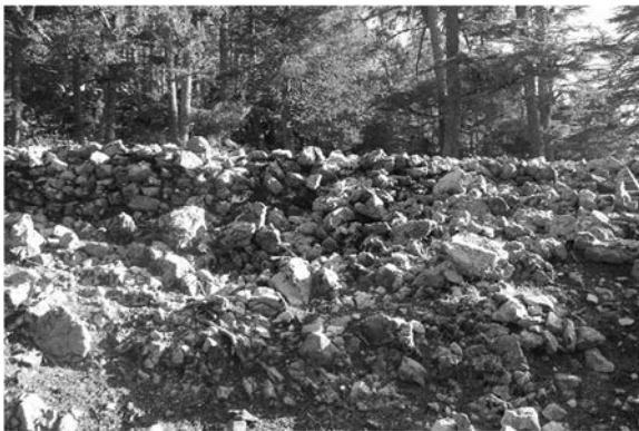
Fig. 26) Retaining walls of the road at Duman Pass.
