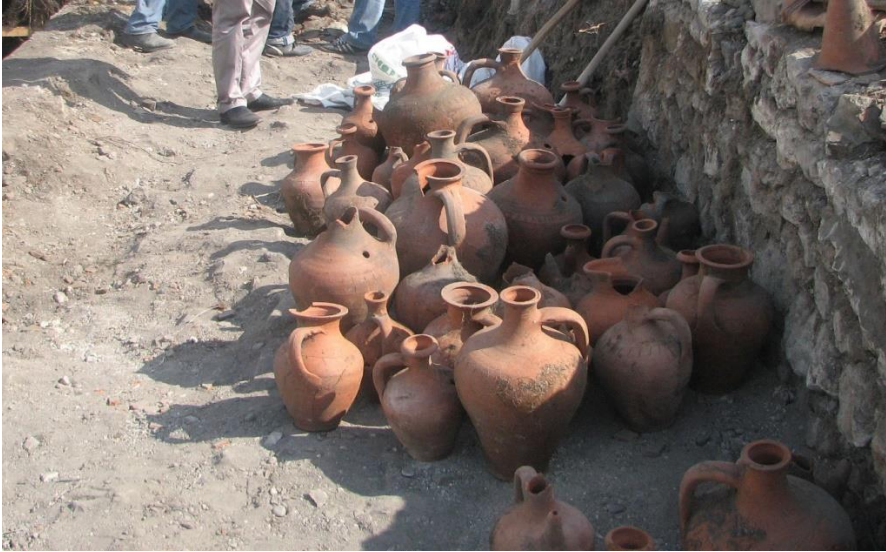
Figure 3: Some of the pottery vessels used as fill material in the roof of Alaca Han
