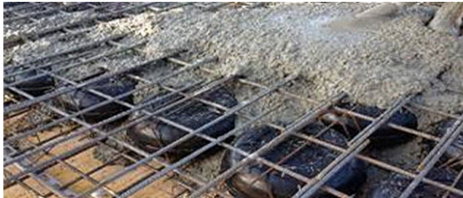
Figure 7. Concreting on Cobiax modules [11].
