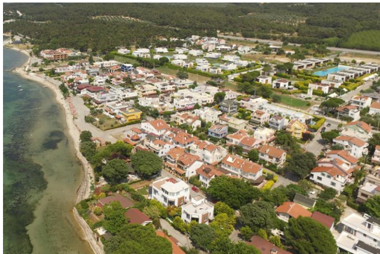
Figure 5. General Facade Views (Original. 2023)
