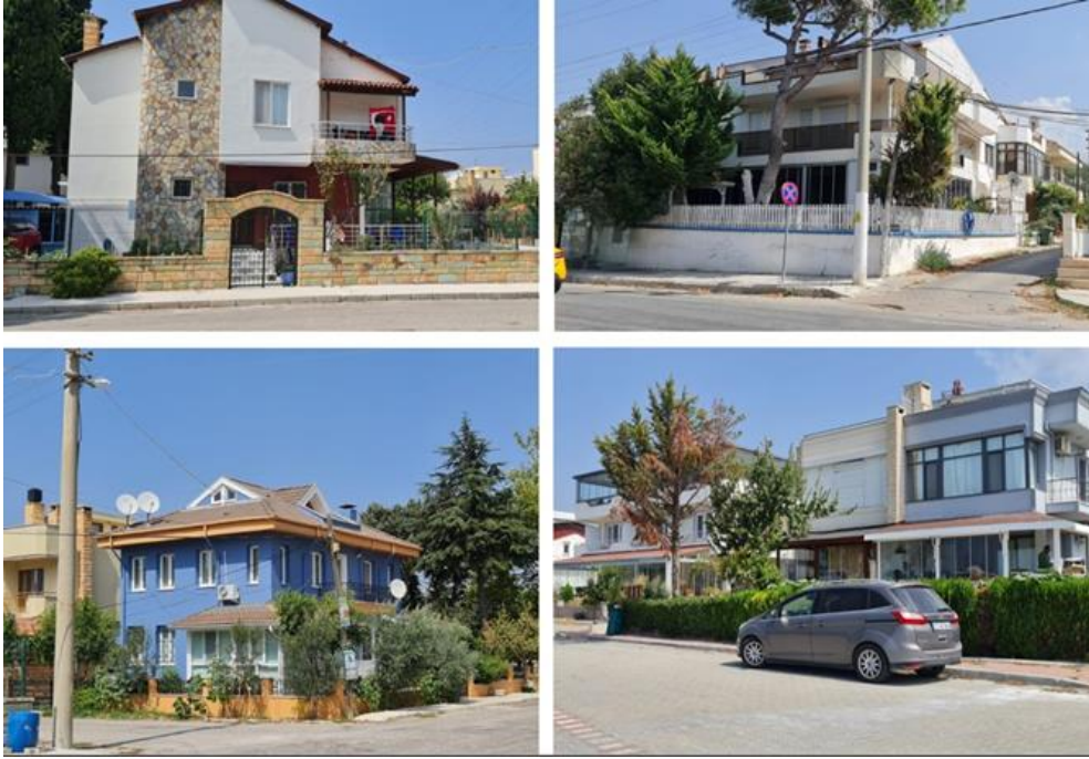
Figure 6. Facade Views (Original. 2023)
