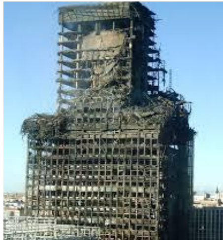
Figure 7. As a result of a fire that started in the electrical shaft in the Windsor Tower [25].
