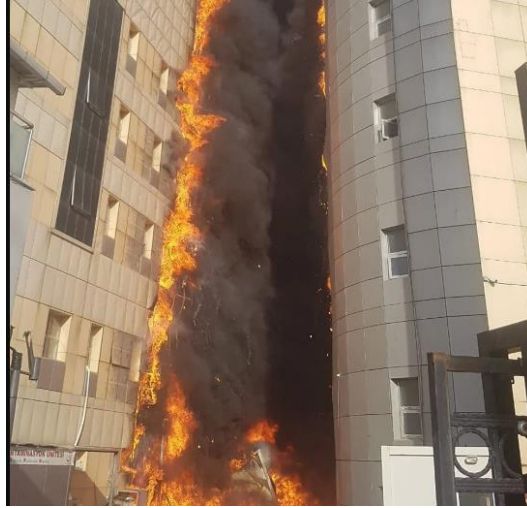
Figure 2. The growth of the fire that started in the waste storage area [11]
