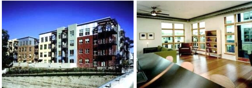
Figure 1. ERD Building; MIDTOWN LOFTS, Minneapolis (Url-1)
