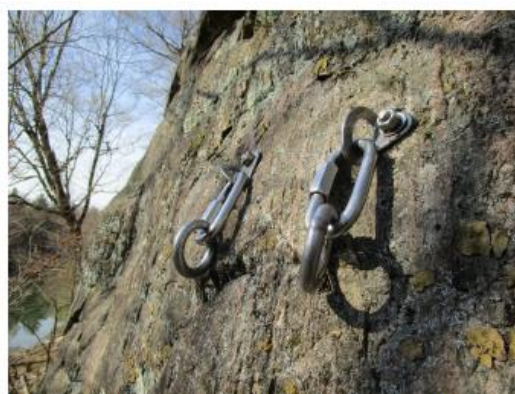
Figure 4. Expansion bolts with quick links and steel rappel rings.
