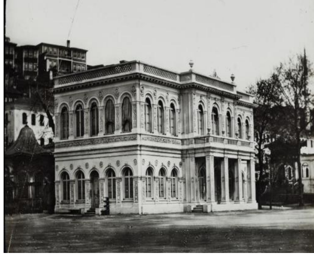
Fig. 22. Tophana Pavilion East View, near Tophana Fountain 91
