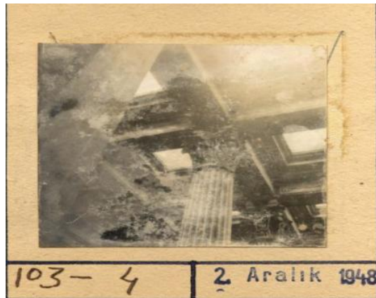
Fig. 17. First Floor Natural Light Installment on the Waffle Slab Ceiling and Corinthian Style Columns 80
