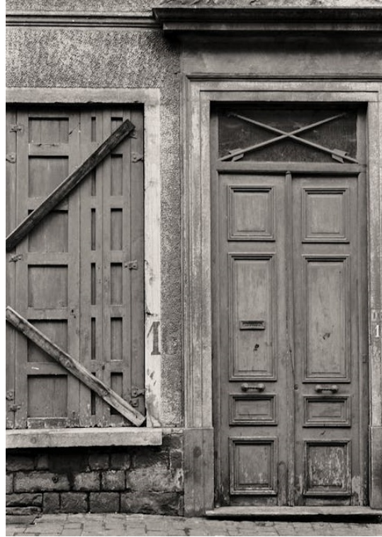
Figure 3. Use of wood in door and window (Codden, 2024)
