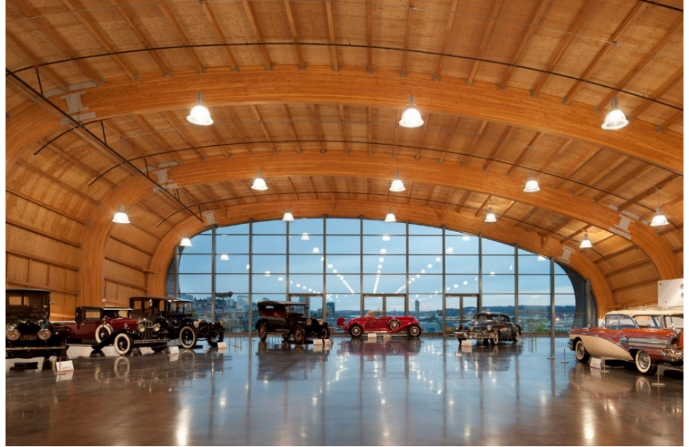
Figure 5. GLT beam and plywood ceiling cladding - LeMay Museum, Tacoma / ABD (LeMay Museum / LARGE Architecture, 2024)
