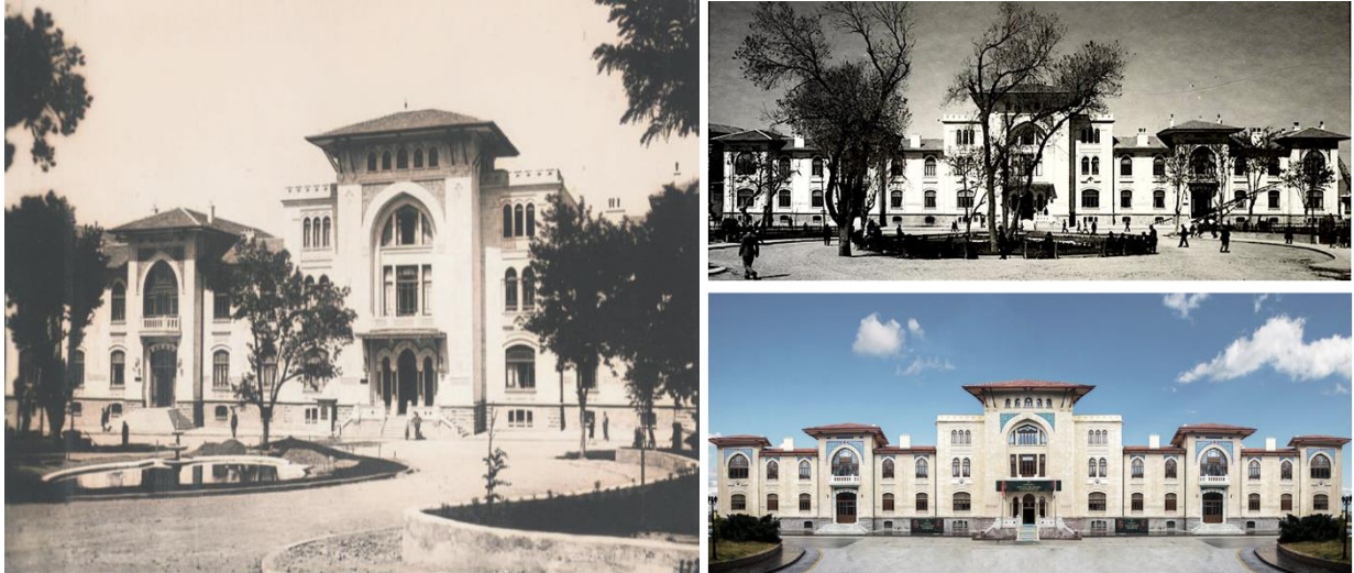
Figure 4. The Old Prime Ministry Building in Ankara, Salt Research, Ülgen Family Archive (on the left); https://www.asbu.edu.tr/tr/genel-bilgi (on the right)[19]
