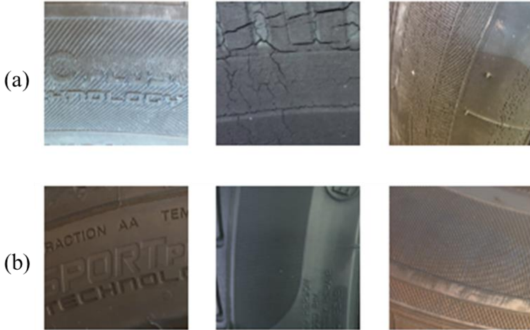
Figure 3.2. Sample tire images, a) Cracked and b) Normal.
