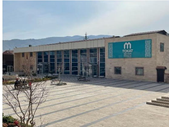
Figure 2. Tokat City Museum Entrance (North) Facade (S. Seyfi, 2024).
