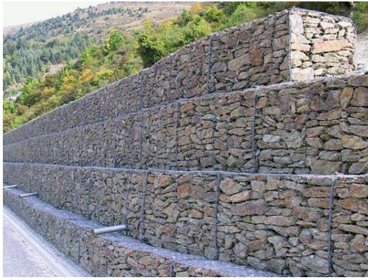
Fig.14 Gabion-retaining wall
