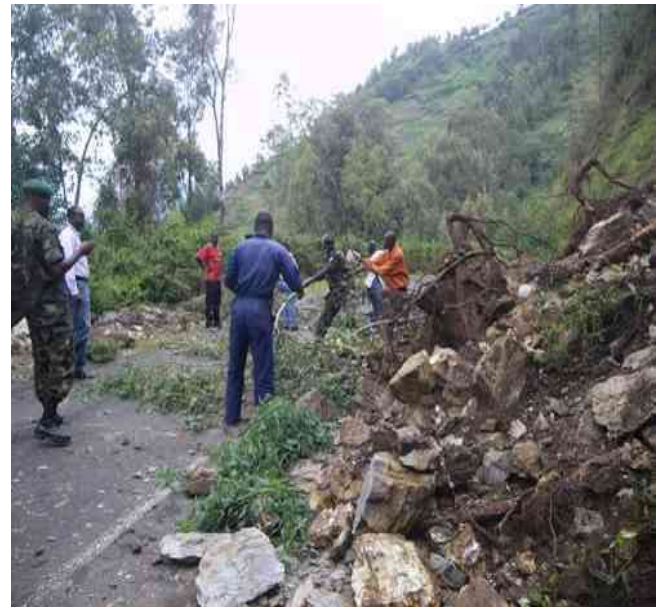
Fig.7 Landslides caused by manmade works (Roads), Ngororero and Rubavu, REMA 2013
