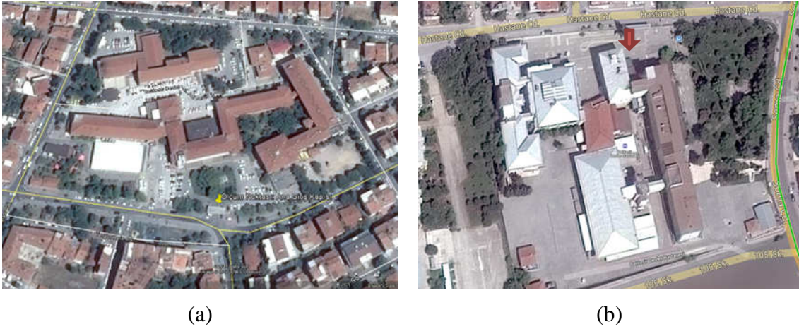
Figure 1. Balıkesir state hospital (a) and Atatürk state hospital (b).
