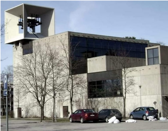
Figure 12 (up-left). Järvenpää Church in Finland (Architectural Uprising, n.d.-j)
