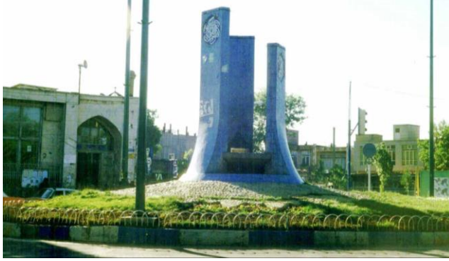
Figure 2. The destroyed square and mosque in Āli Qāpu (Source: شهردار از عکسهایی و قدیم اردبیل (n.d.). Retrieved April 01, 2016)
