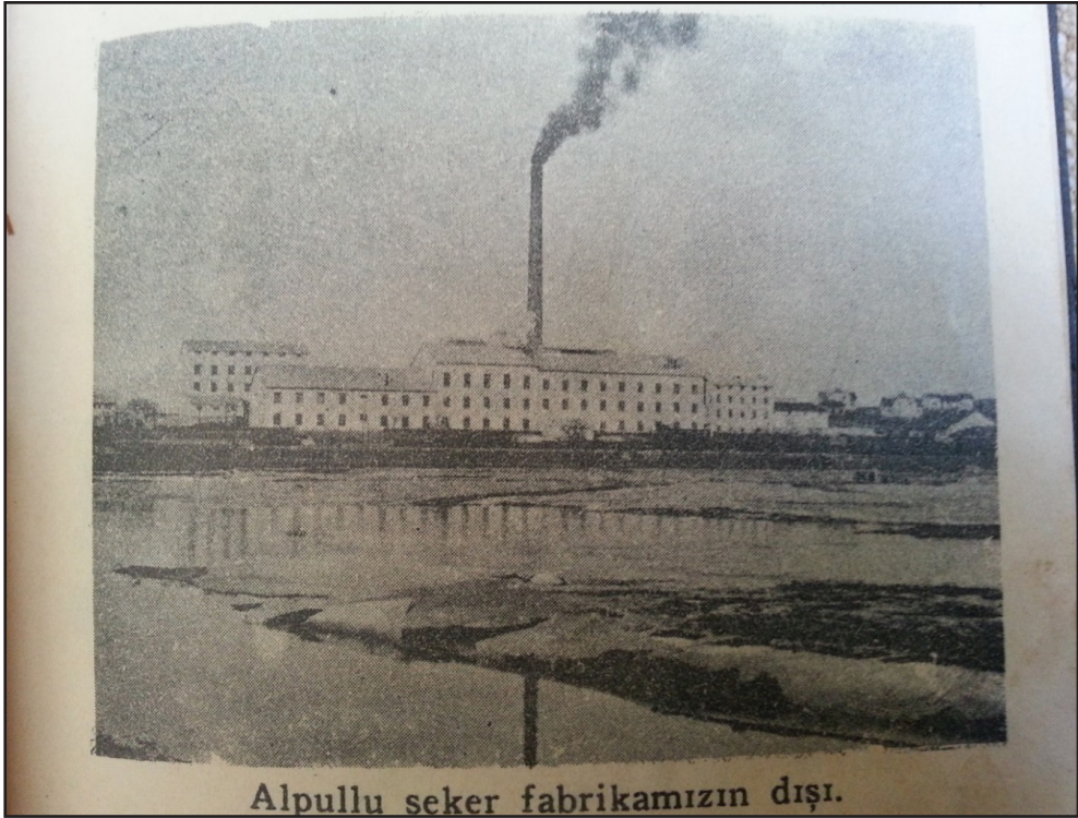
Photograph.1. Outer side of Alpullu Sugar Factory
