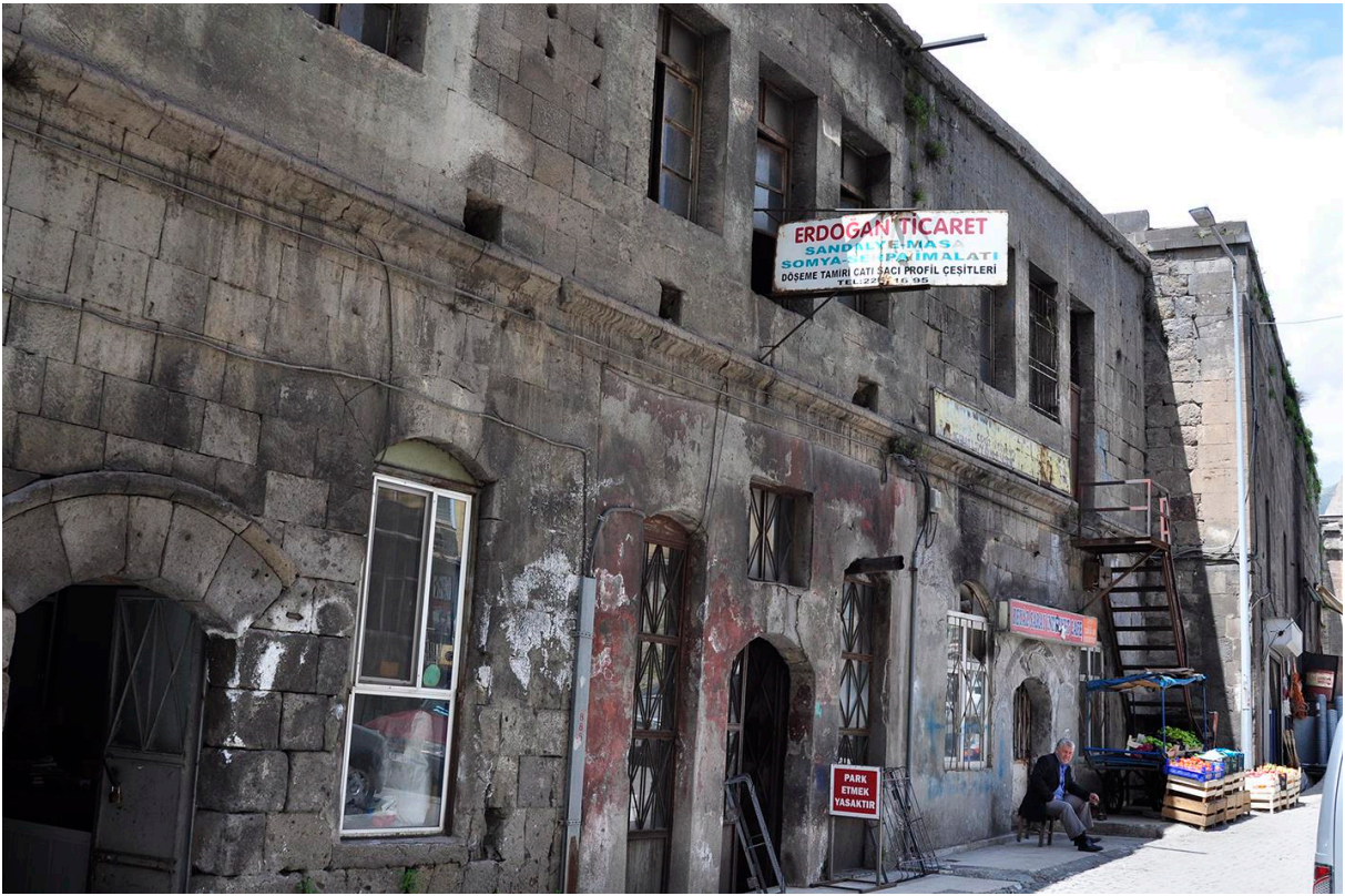
Figure 9: Eastern façade of the qaysâriyya and madrasa.
