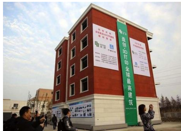
Fig.8. World’s first 3-D printed apartment building by Win Sun, 2015, Source: retrieved July 9, 2015 from http://www.cnet.com/pictures/3d-printed-apartment-building-and-mansion-pictures/
