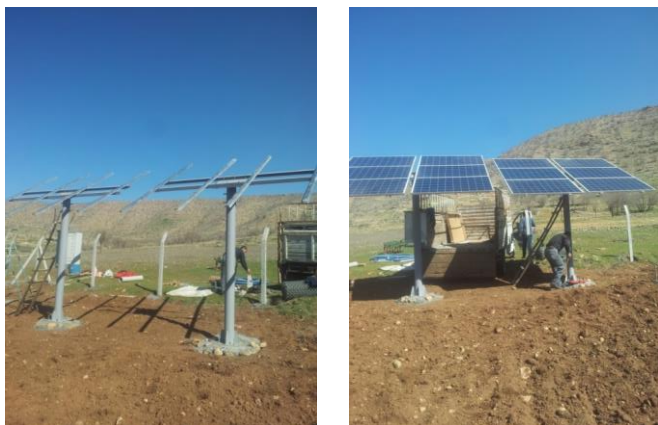
Figure 9. Installation of photovoltaic system in the field
