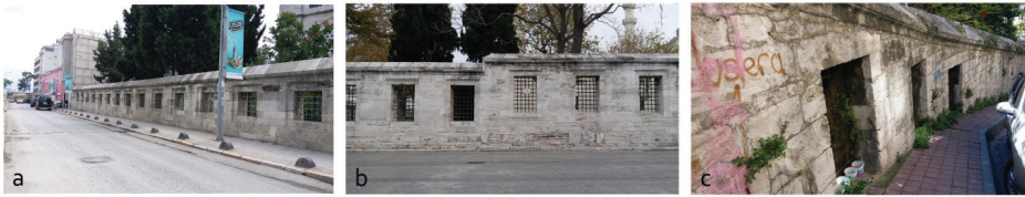
F. 6. The coping formation; a) the eastern surrounding wall of the Kılıç Ali Pasha Mosque, b) the western surrounding wall of the Süleymaniye Mosque, and c) the eastern surrounding wall of the Kadirga Sokullu Mosque (Sources: Author, 2018)
