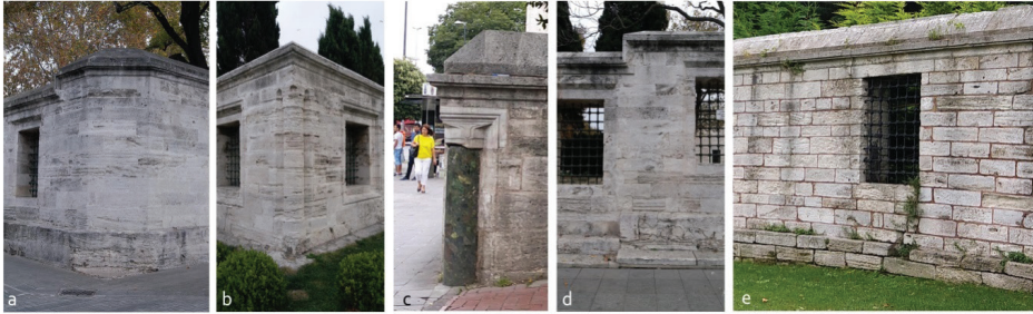
F. 5. The corner turns ( çal köşe ); a, b) Süleymaniye Mosque, c) Şehzade Mehmed Mosque, and the wall base ( duvar pabucu ); d) Süleymaniye Mosque' west surrounding wall, e) Şehzade Mehmed Mosque's north surrounding wall (Author, 2018)
